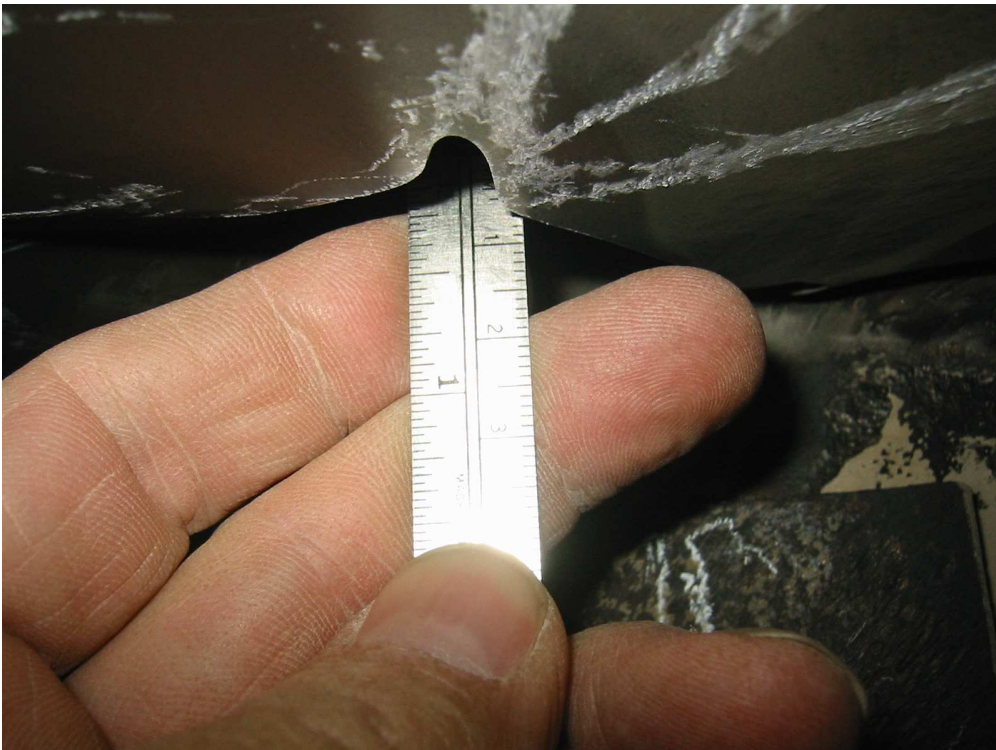
Cold end spool erosion damage
