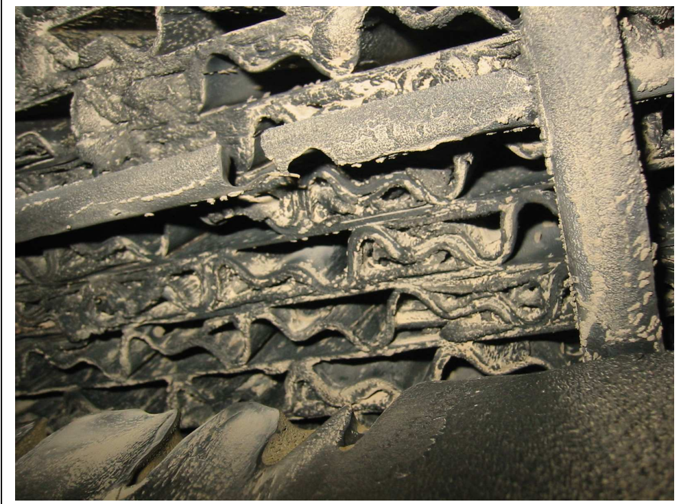
Cold end element pluggage, basket bar erosion and grating erosion
