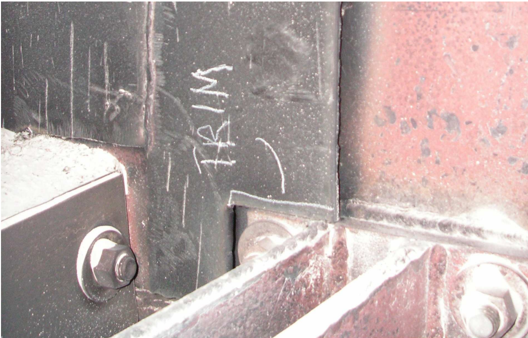
Static seal bottomed out against the sensor support
