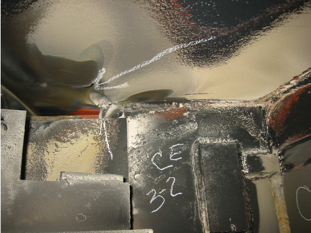
Cold end spool erosion damage
